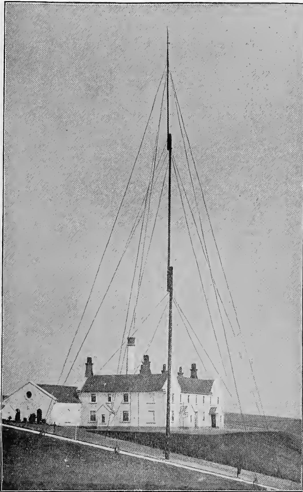
FIG. 50 (Fig. 1, p. 7, The Electrician , Vol. XLIII.)—Mast at South Foreland, from which Signals went to a similar Mast at Wimereux, near Boulogne.
